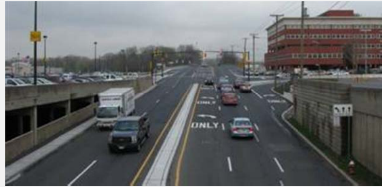
Looking north along Maywood Avenue
